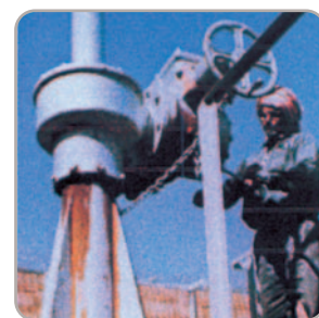
The first actuator built by EIM was installed on this pipeline in Saudi Arabia in 1949. It continues to give reliable service today—despite metal temperatures that frequently reach 170°F (77°C).
