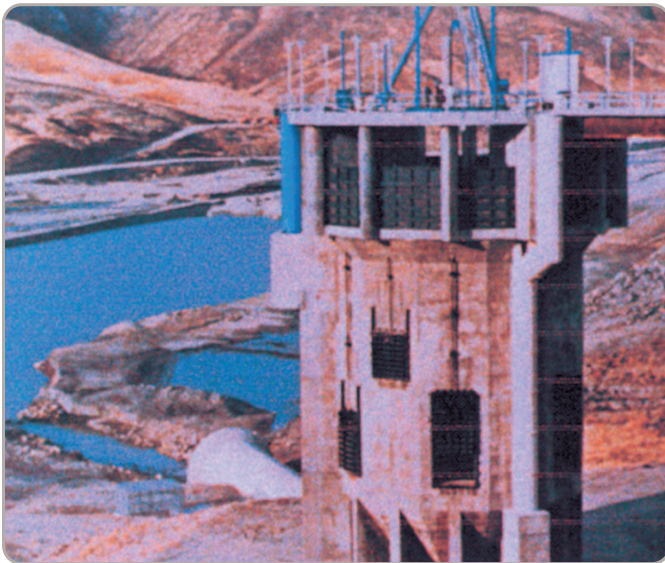
You'll find EIM wherever the going is tough. EIM actuators open and close sluice gates in this water project near Los Angeles.
