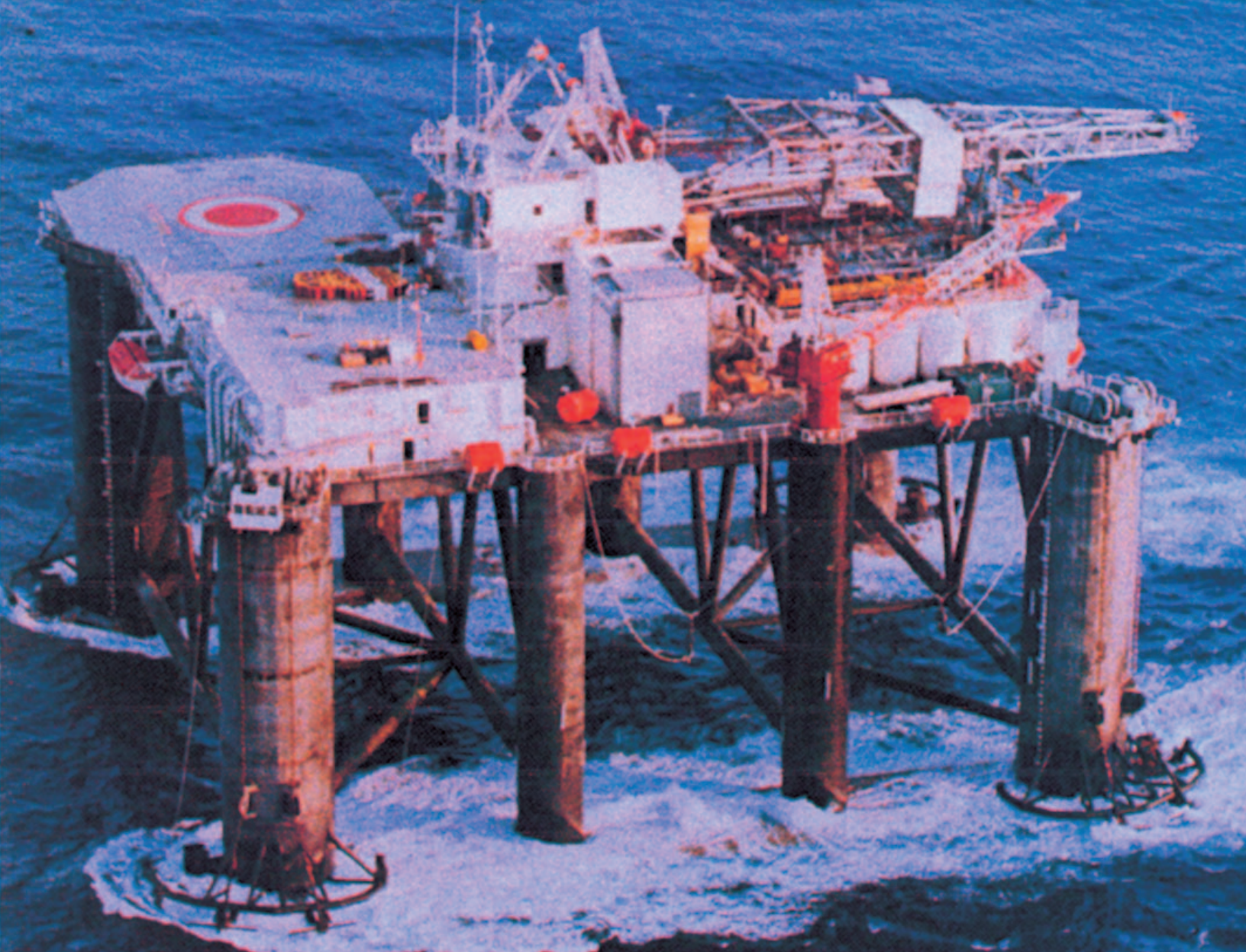
This portable drilling tower in the North Sea uses EIM electric actuators to control flooding and emptying of ballast water tanks in the tower legs.
