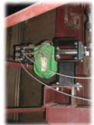
Burner Nozzle Tilt Drives
